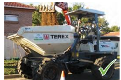
Tipping spoil directly into a truck or skip avoids stockpiling
