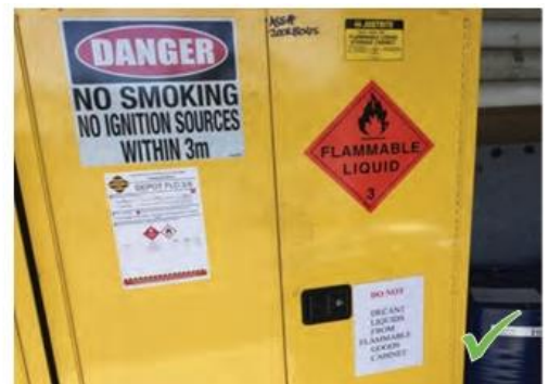
Use bunded chemical storage cabinets to store fuels and chemicals
