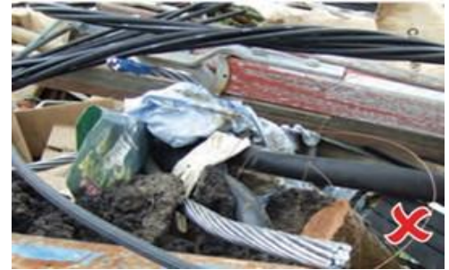
Example of poor waste segregation
