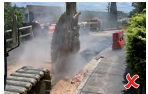
Prevent dust from leaving the worksite
