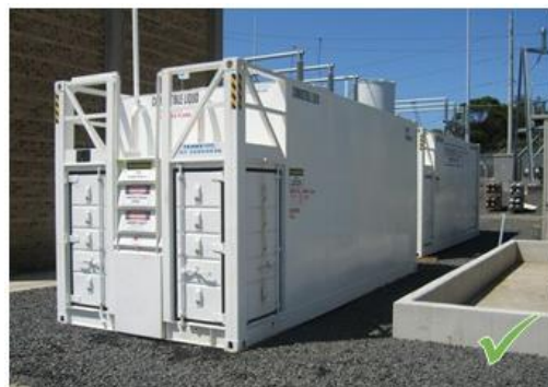
Self-bunded (double-walled) portable tanks can be used for permanent storage
