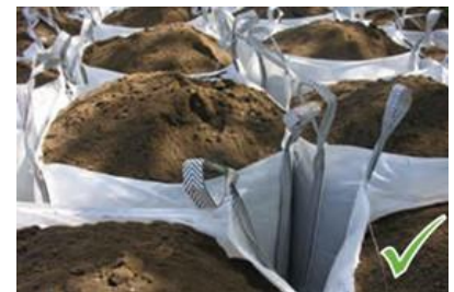
Bulk storage bags help contain materials
