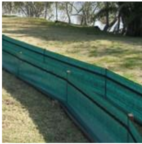
Figure 2.1-2: Sediment fence installation instructions
