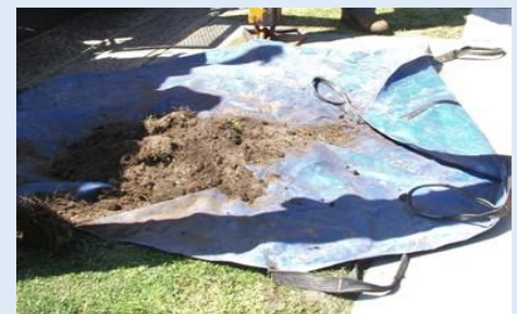
Spoil temporarily placed on tarp to contain spoil and assist clean up
