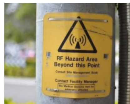
Example of identifier plate located near an RF transmitter
