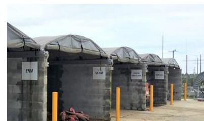
Store material in correct bays to avoid cross contamination
