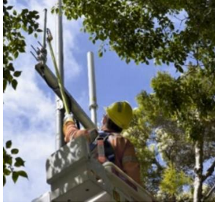
Testing the antenna
