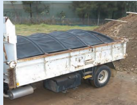
Cover loads to prevent dropping spoil or creating dust
