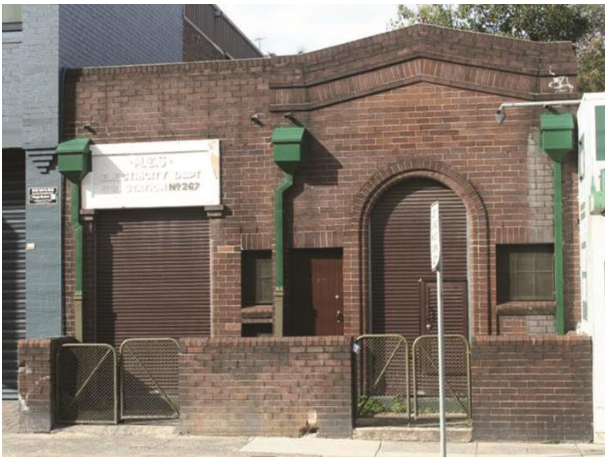
Ausgrid S170 heritage substation. Also, Local heritage
