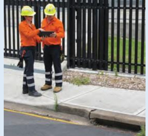
Locating slopes, drainage lines and inlets will help determine the controls required
