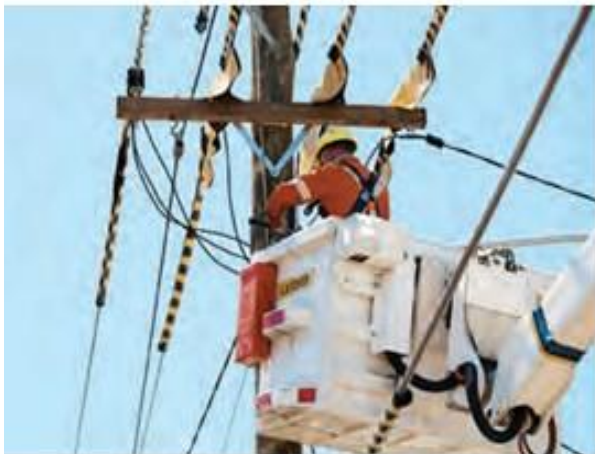
Live line work
