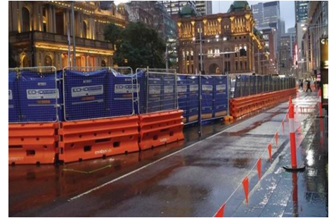
Portable noise screen used to mitigate noise
