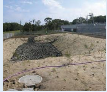
Rehabilitate disturbed areas to prevent erosion
