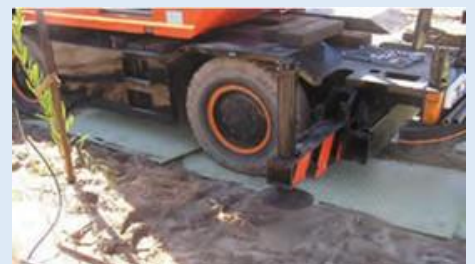
Temporary construction mats help minimise ground disturbance
