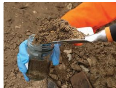
Spoil from below the slab should be assumed SCW unless tested otherwise
