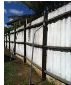
Distribution substation fence
