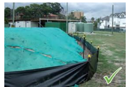
Stockpile covered to prevent dust and a sediment fence used to filter run-off
