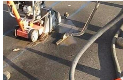
Wet-vac used to collect saw-cutting slurry
