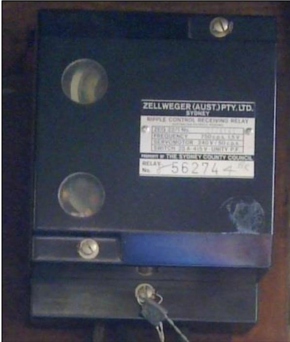
Figure A1: Ripple Receiver
