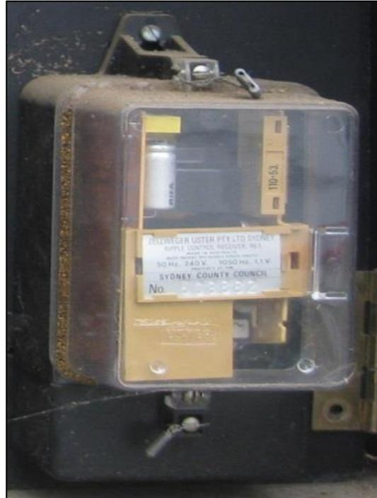
Figure A2: Ripple Receiver
