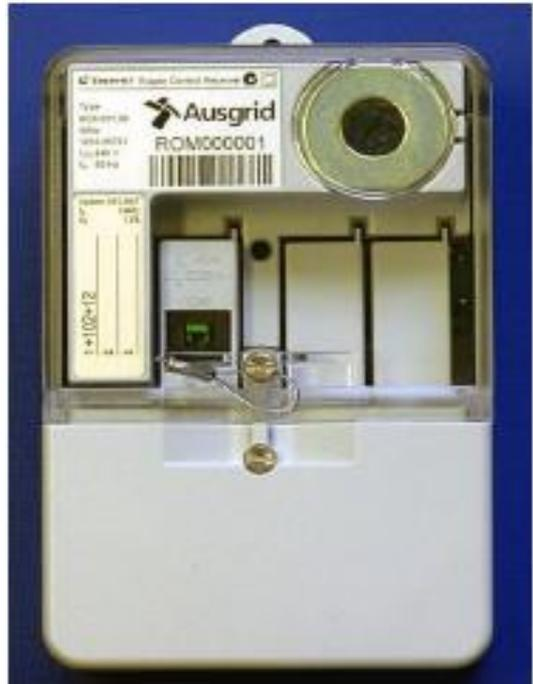
Figure A4: Ripple Receiver
