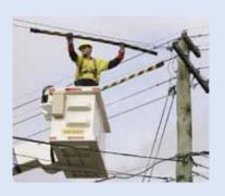
Field crew makes the site safe, isolates the affected area and restores power to as many customers as possible before commencing repairs.
