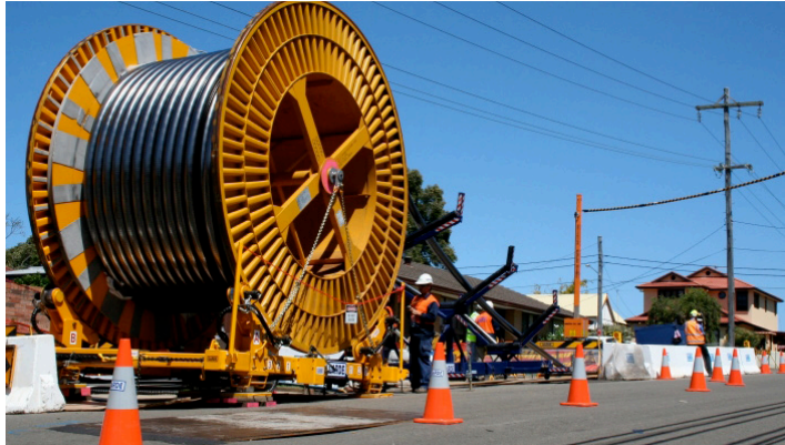
Cable installation on a similar project
